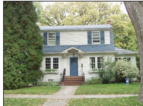
209 Bedford Avenue (Colonial Revival, second period)
